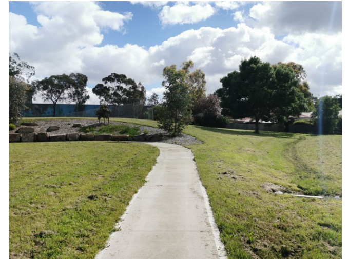
figure 6 Existing accessible path and drainage channel
