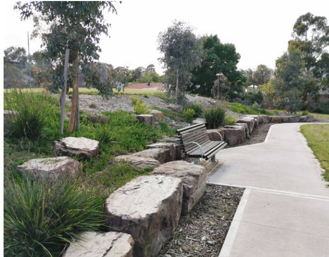
figure 4 Stone retaining wall and planted embankment
